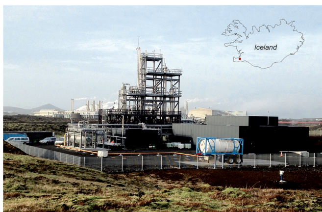
Figure 1. The “George Olah Carbon Dioxide to Renewable Methanol Plant” of Carbon Recycling International in Iceland based on local geothermal energy. The first commercial carbon dioxide recycling plant operating in the world (Courtesy: K. C. Tran, CEO, Carbon Recycling International, Iceland).
